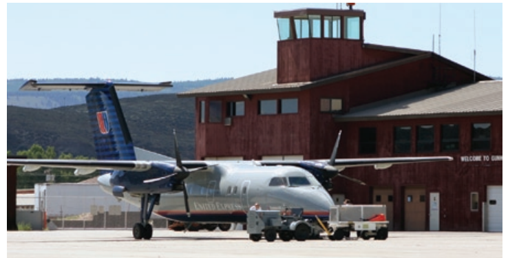
Gunnison-Crested Butte Regional Airport-Gunnison, CO
